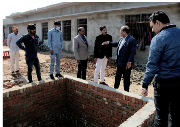
Dy. Director, I/C S.O. Lucknow Shri D.S. Bhati inspected under construction CFC by Hand Knotted Carpet SFURTI Cluster at Mirzapur.
