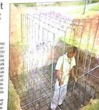
Work on the installation of the charkha begins on the riverfront
